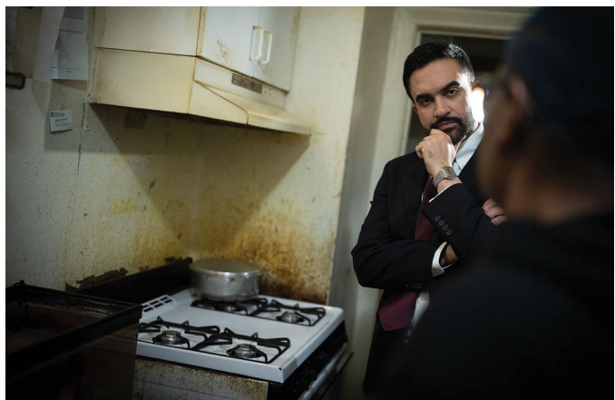
Mayor Mamdani inspects a New York apartment for mold, lead paint, and other hazards, 2026. (Photo: Michael Appleton, NYC Mayor's Office)
