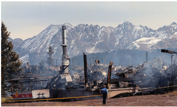
Smoldering ruins of Vail Mountain's Two Elks restaurant on Oct. 20, 1998, after a fire—later claimed by the Earth Liberation Front—caused $12 million in damage at the ski resort. (AP Photo/Jack Affleck)
